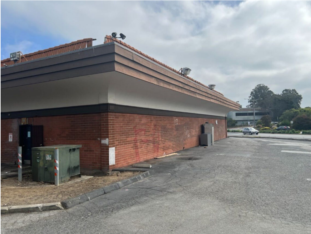
Photograph 3: Overview from western corner of the project area. Viewing east.
