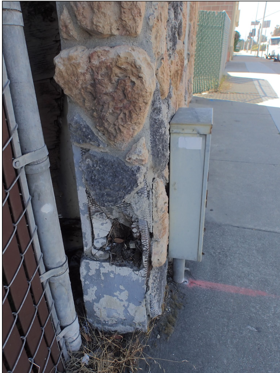
214 Airport Boulevard, west façade. Close up of faux masonry cladding. View south. September 20, 2018.
