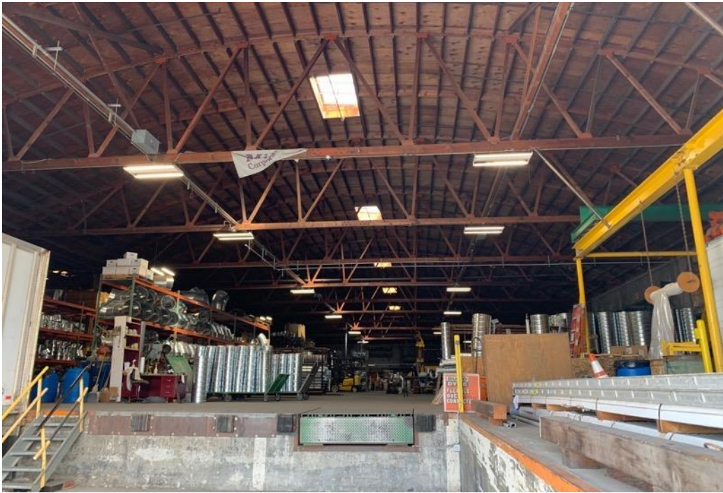
Figure 24. 145 Sylvester Road. Interior view of warehouse showing wood frame roof trusses and loading bay, looking east.
