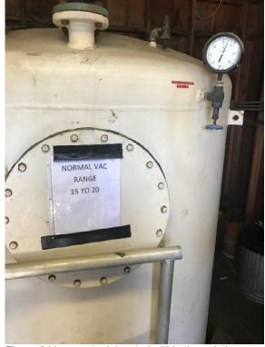
Figure 2 Vacuum tank located within the existing pump house.
