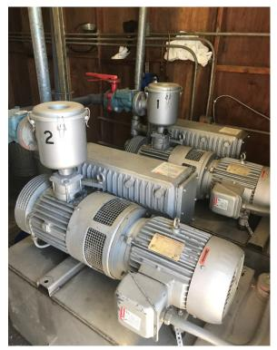
Figure 1 Existing vacuum pumps located within the pump house.
