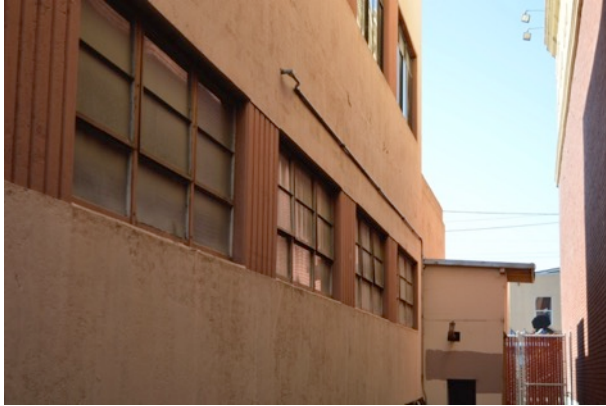
Figure 18. Steel windows located along first story of the west elevation. Shed roofed addition pictured in background, looking south.
