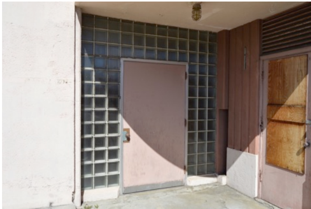
Figure 13. Flush wood door surrounded by prismatic glass block, at east elevation. Partially boarded-over flush wood door at south elevation pictured at right, looking northwest.
