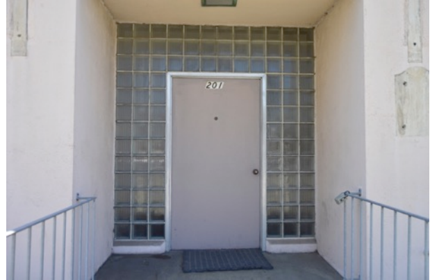
Figure 6. Recessed entrance with flush-wood door and glass block surround at facade, looking south.
