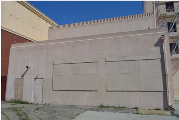
Figure 15. Infilled and boarded-over door and window openings at west end of south elevation, first story. Standard replacement windows at second story.
