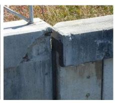
Due to the high volume of Average Daily Traffic (ADT), full closure of the bridge may not be allowed and temporary traffic control measures will be implemented to allow the public to safely travel across the bridge. The scope of work includes replacing the existing joint seals. There is a concrete curb median on the bridge which crosses over the joint seal. In order to replace the joint seals. The concrete median will be removed and reconstructed after replacing the joint seals.
