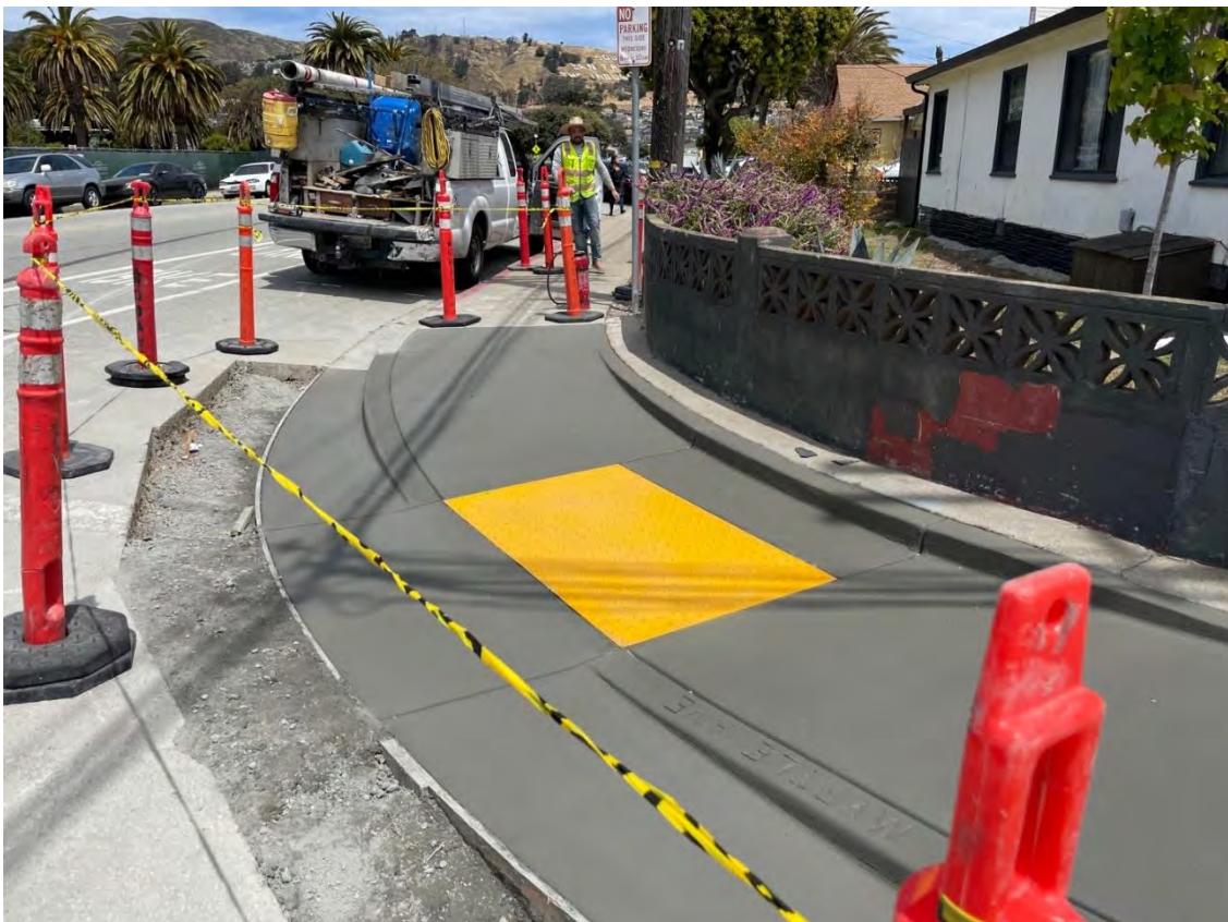
Photo 8: Construction of curb ramp at W Orange Ave and Myrtle Ave
