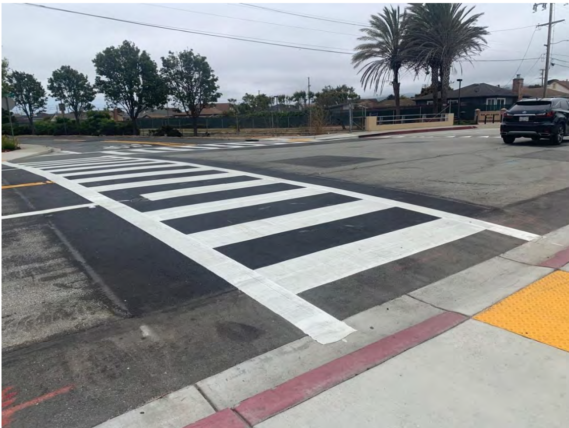
Photo 6: Completed High Visibility Crosswalks at W Orange Ave and N Canal St
