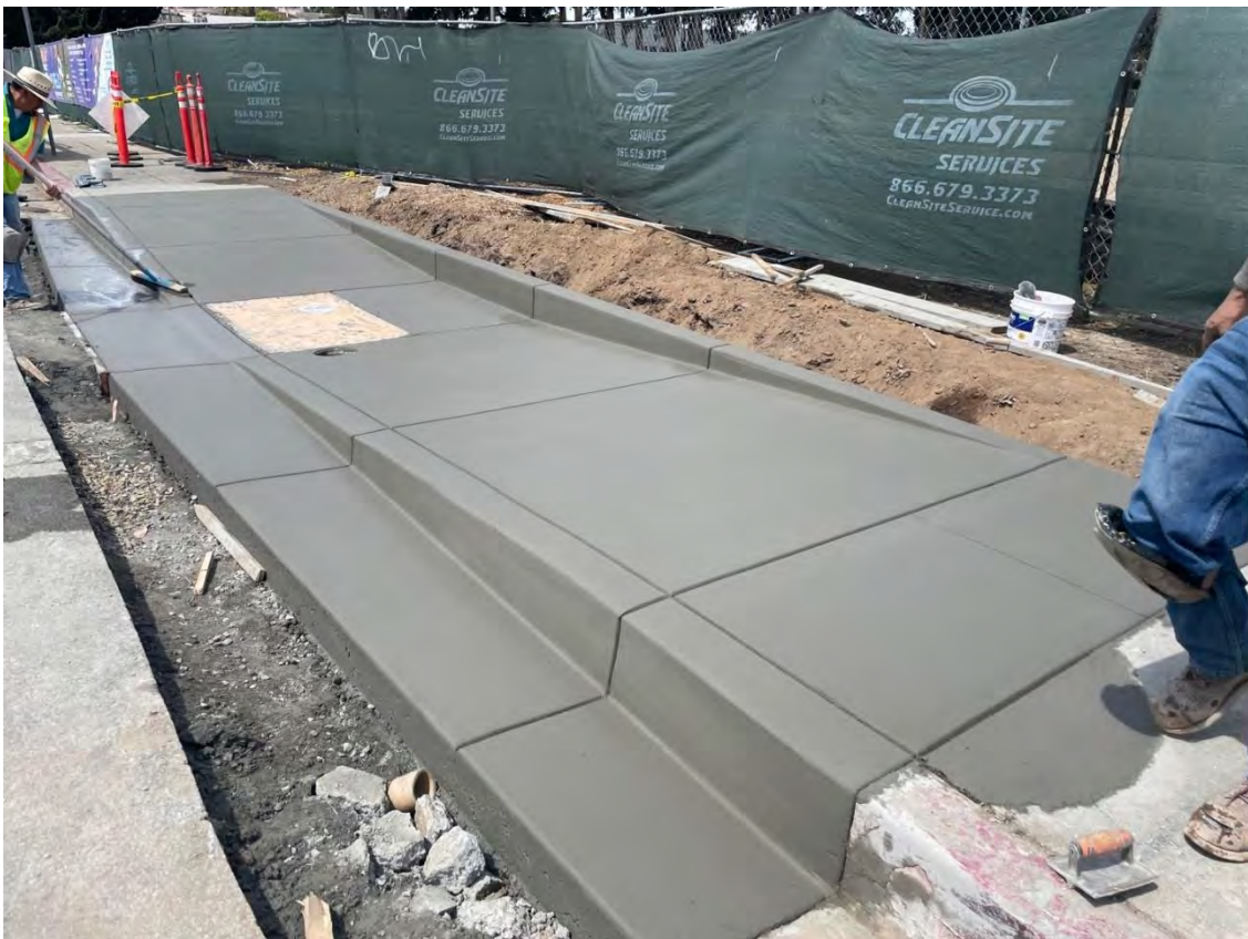
Photo 10: Construction of curb ramp at W Orange Ave and Myrtle Ave
