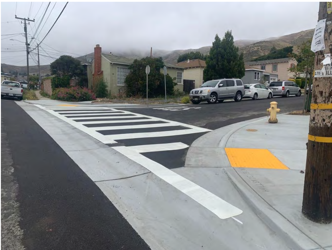
Photo 2: Completed Curb Ramp and High Visibility Crosswalks at Hillside Blvd and Claremont
