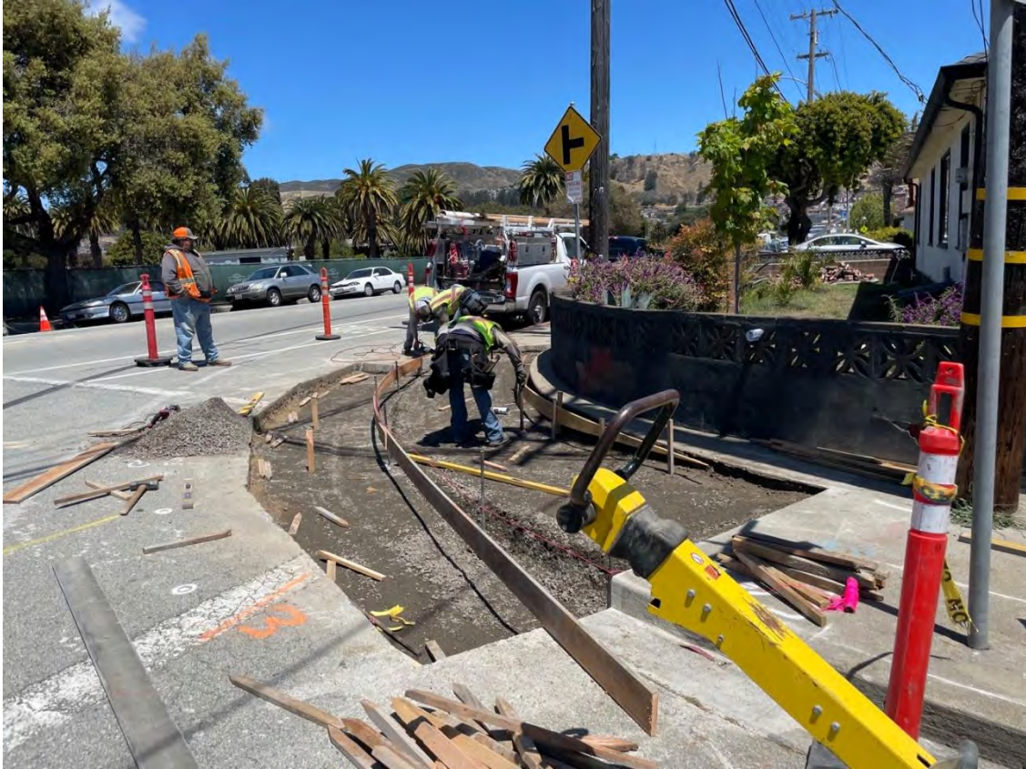
Photo 7: Construction of curb ramp at W Orange Ave and Myrtle Ave
