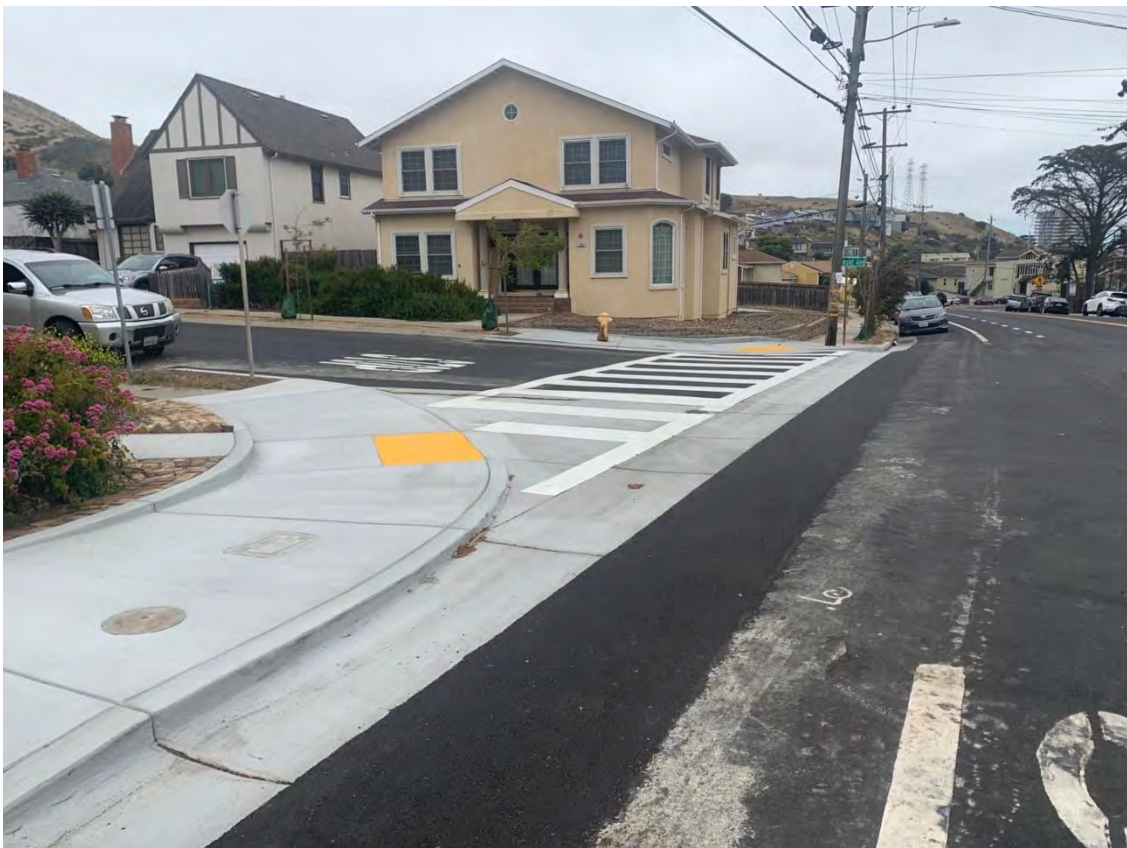
Photo 4: Completed Curb Ramps and High Visibility Crosswalks at Hillside Blvd and Claremont Ave
