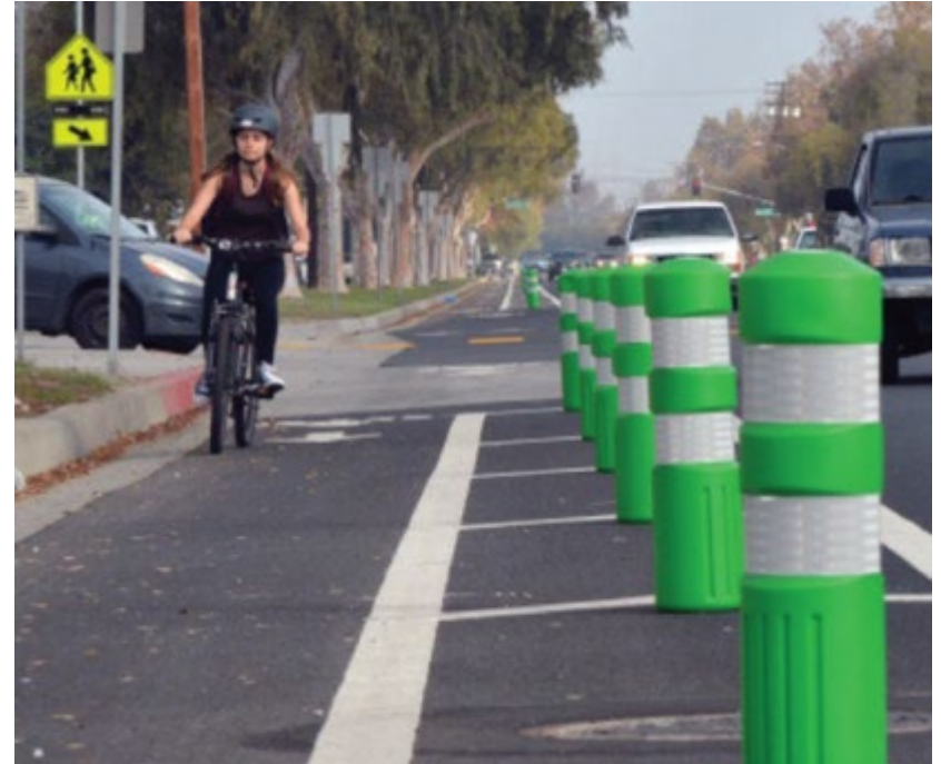
K-71 bollards (Source: Google Maps)
