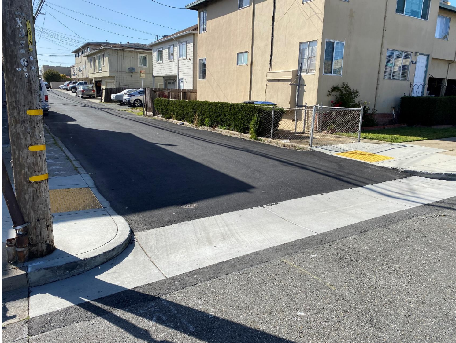
Third Lane facing West / Rubberized Chip Seal (after to Surface Seal)
