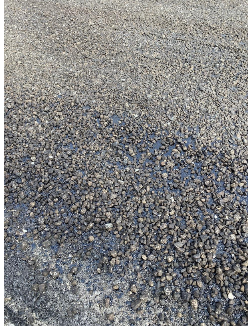
Third Lane facing West / Rubberized Chip Seal (prior to Surface Seal)
