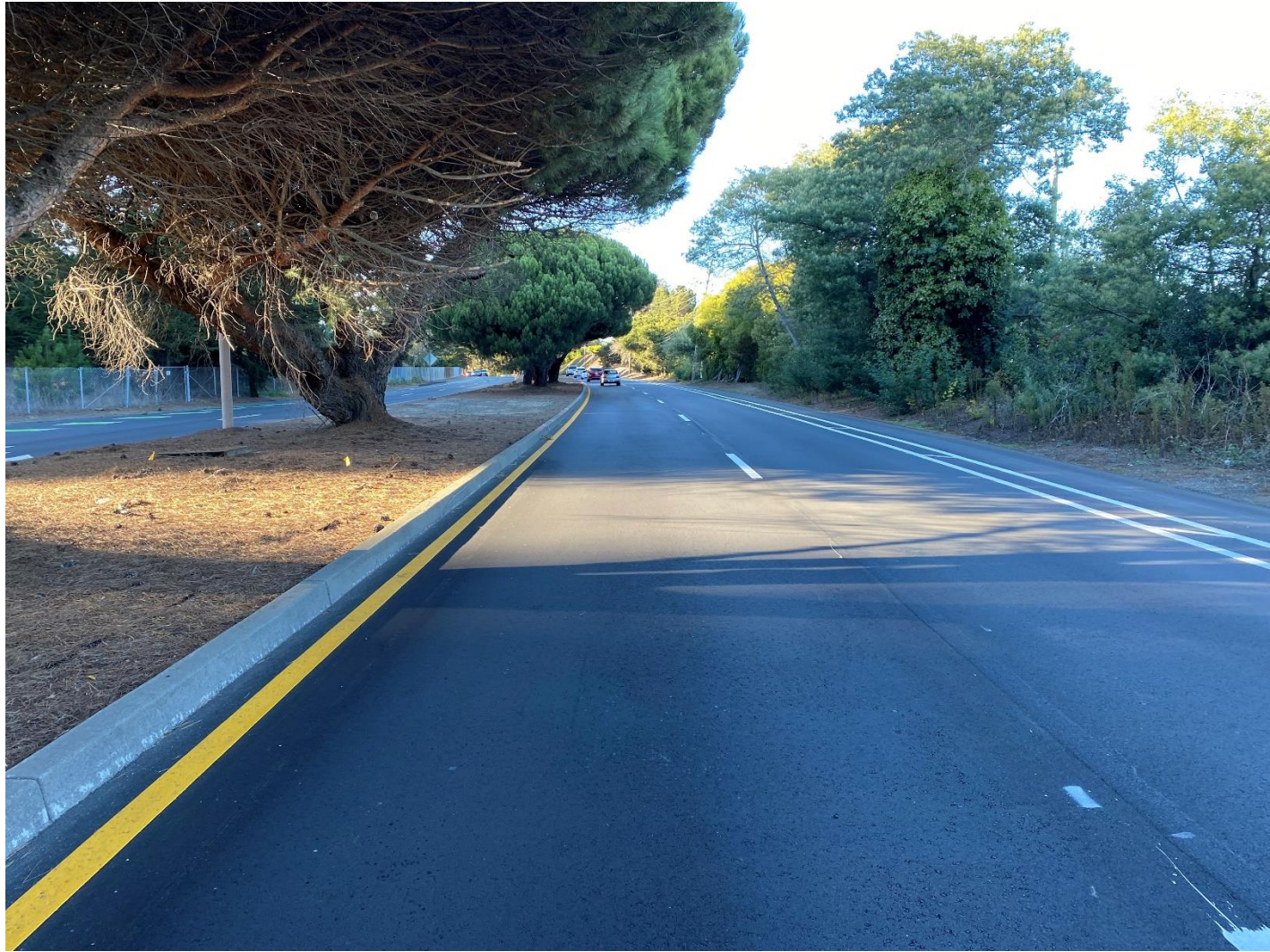
Junipero Serra Blvd near Avalon facing Northbound
