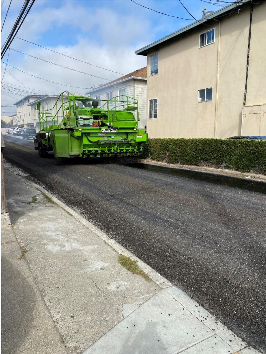
Third Lane facing West / Rubberized Chip Seal (prior to Surface Seal)
