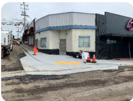
Figure 6 – City of South San Francisco OBAG 2 Street Rehabilitation
