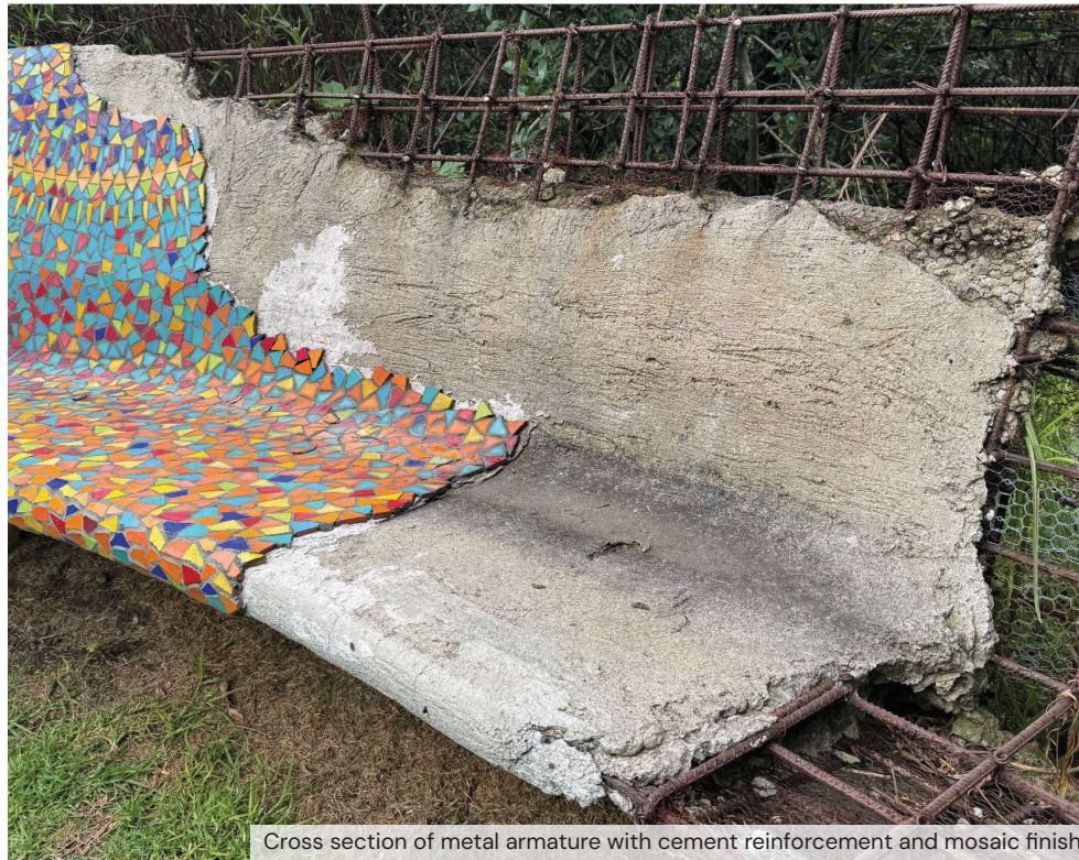
Ferrocement sculpture, smoothing & detailed shaping
