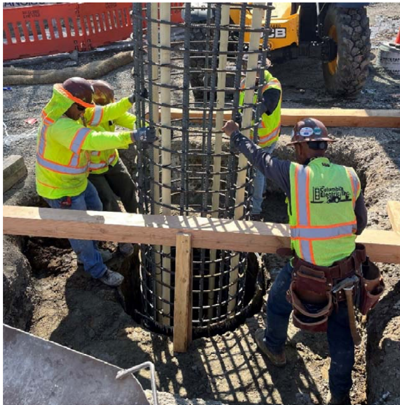
Photo 8: Installation of the rebar cage for the traffic signal foundation
