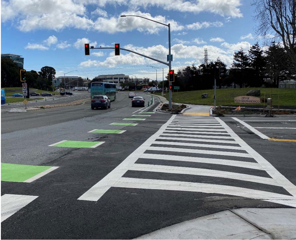
Photo 11: Installation of new dual high-visibility crosswalk and bicyclist crossing at the south leg of the E Grand/Grand Ave intersection
