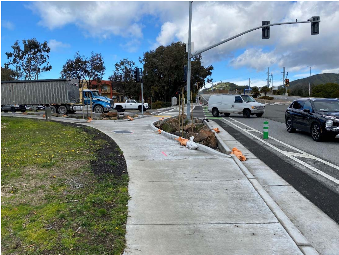
Photo 4: Completion of the new sidewalk and corner extension at the southeast corner of E Grand/Grand Ave
