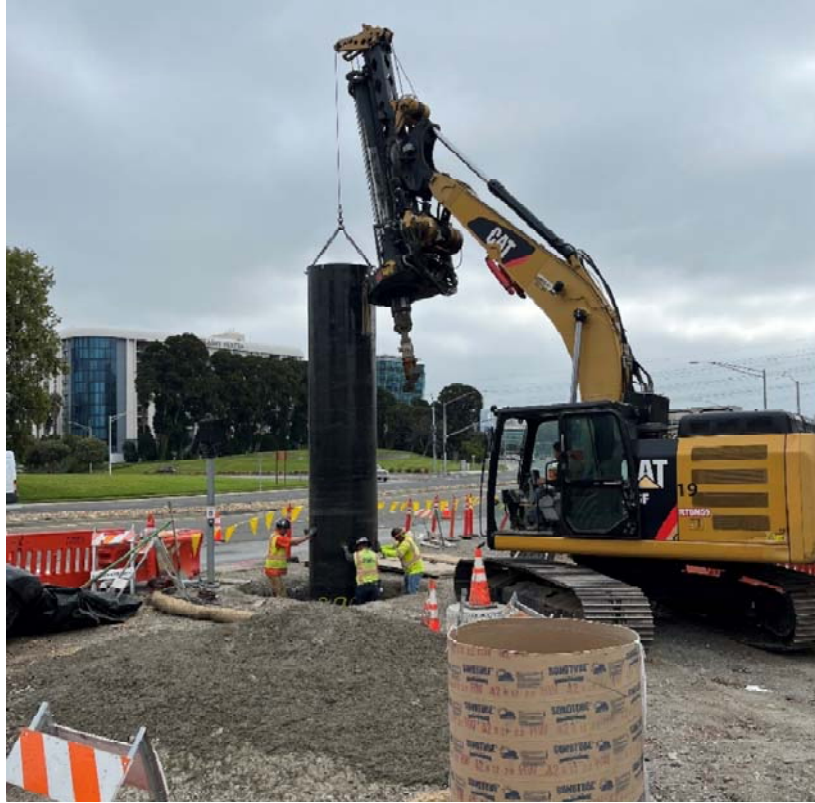
Photo 7: Installation of a steel casing for the traffic signal foundation
