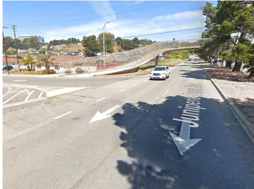
Pedestrian Overhead Crossing at Clay Avenue (Source: Google Maps)
