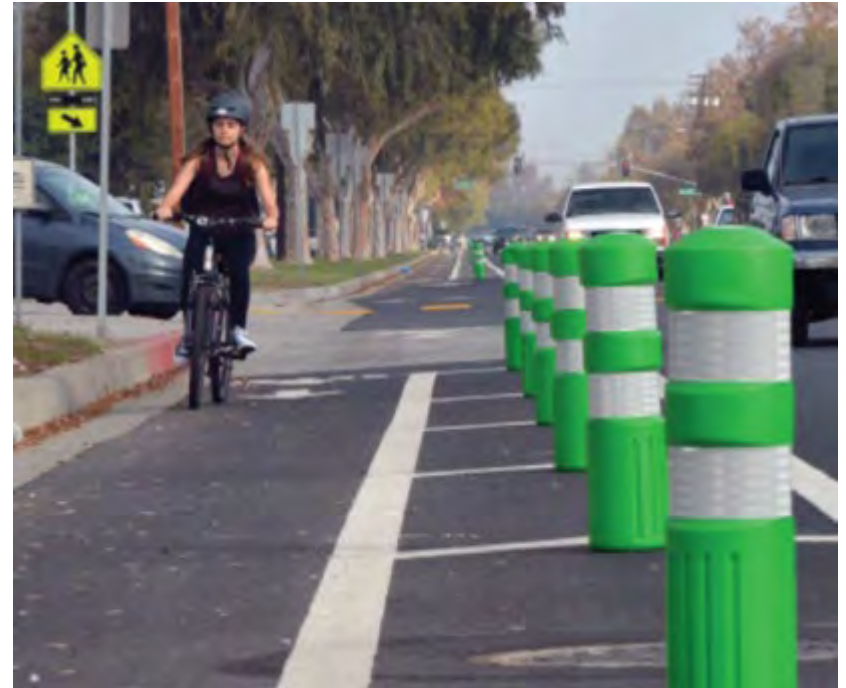
K-71 bollards (Source: Google Maps)
