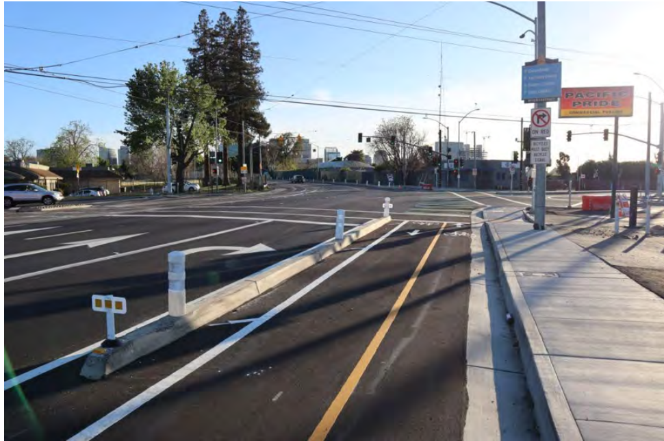
Two-Way Separated Bikeway, N 12 th Street, Sacramento (Source: Google Maps)
