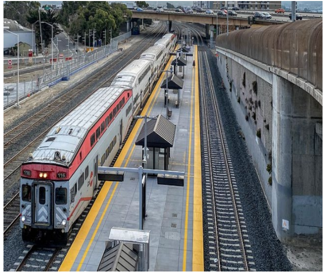
Rendering of the New Widened Central Platform at the South San Francisco
