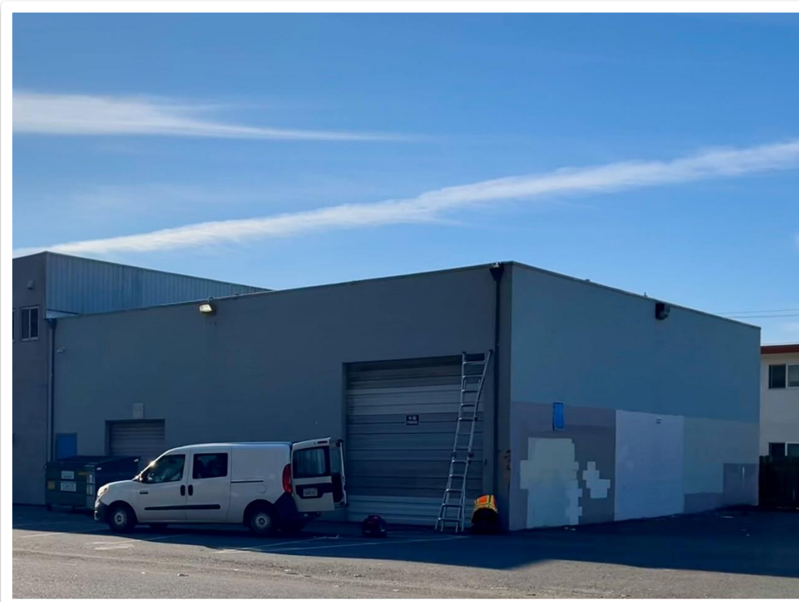
Before (garage used for storage)
