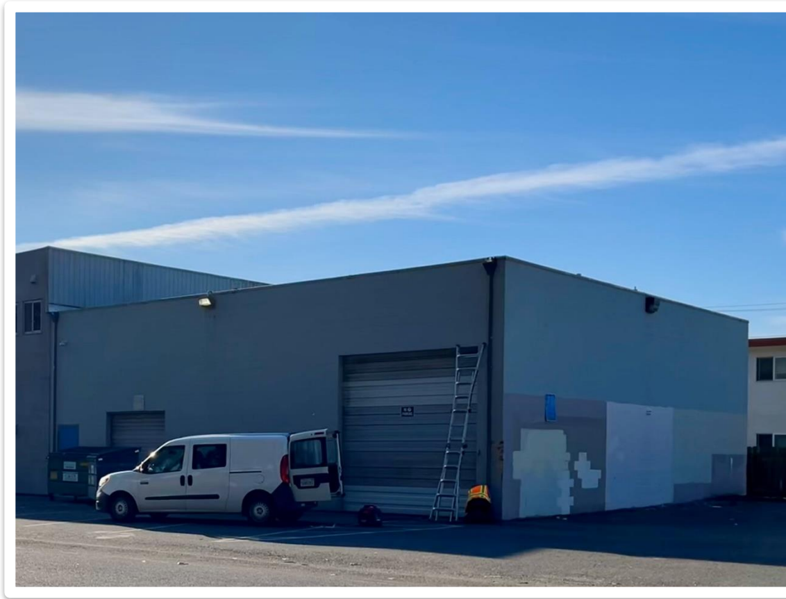
Before (garage used for storage)
