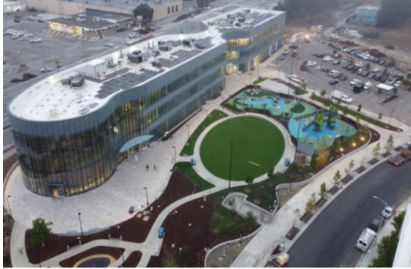
Library | Parks and Recreation Building
