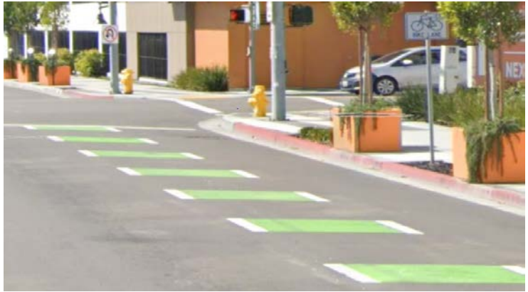
Class II Bike Lane on Airport Boulevard
