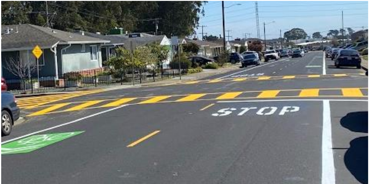
New High Visibility Crosswalks and Advance Line Stop Bars at key school intersections to improve safety for pedestrians crossing the road
