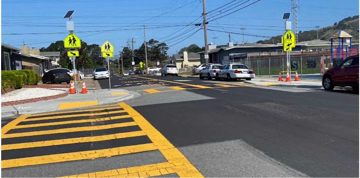
New Rectangular Rapid Flashing Beacons at key school crossings to improve safety for pedestrians crossing the road
