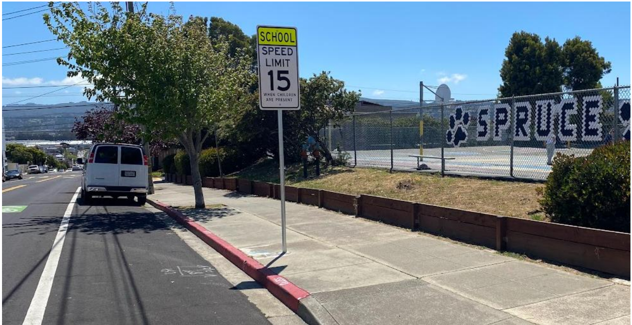
New School Signage and Edge Line Striping at key school corridors to reduce the road width and encourage slower speeds
