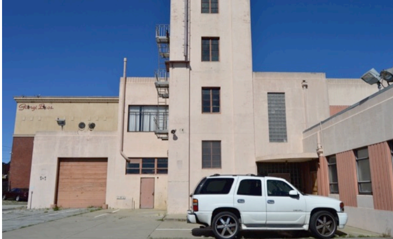
Figure 12. South portion of east elevation with garage bay, drill tower, and rear entrance, looking west.
