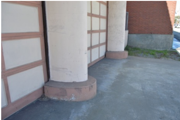
Figure 9. Concrete columns and concrete wheel guards at apparatus bays.
