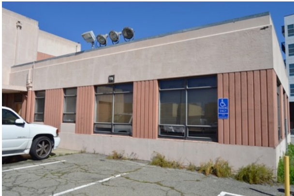
Figure 17. Standard replacement windows at east portion of south elevation, looking north.
