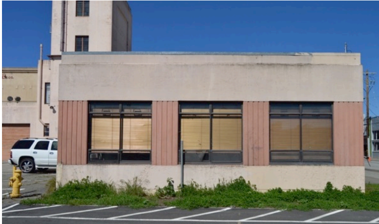
Figure 10. Replacement aluminum windows at north end of east elevation, looking north.
