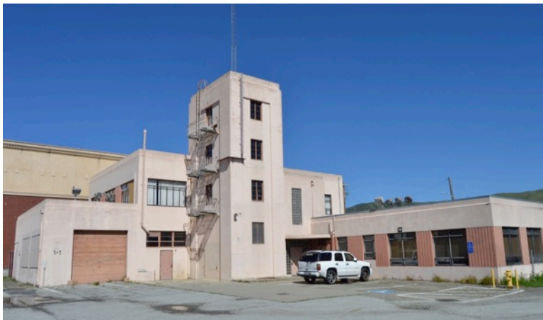
Figure 11. View of east elevation (left) and south elevation (right), looking northwest.
