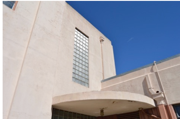
Figure 14. Column of prismatic block glass at east elevation, looking northwest.
