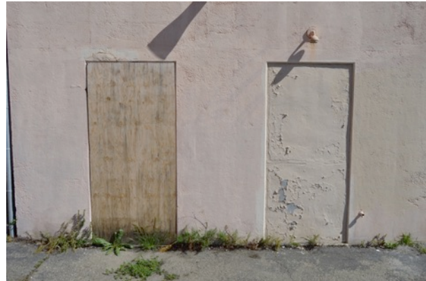
Figure 16. Boarded-over door and infilled door at first story of south elevation, looking north.
