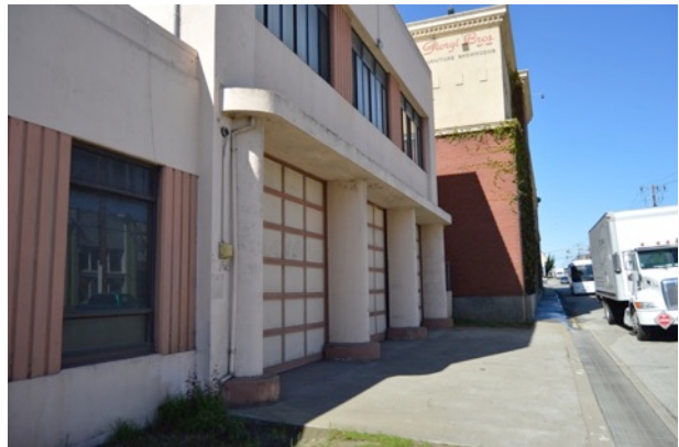
Figure 8. Apparatus bay doors, looking west.
