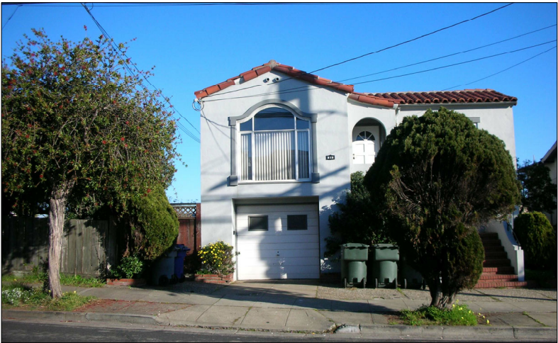
RIGHT-SIDE NEIGHBOR FRONT ELEVATION- A 2 STORY BUILDING.
