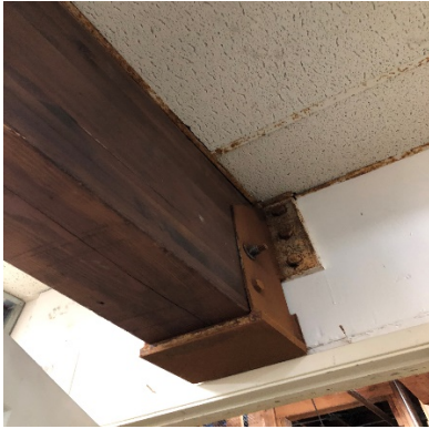
Fig 19 – Retrofit Beam
