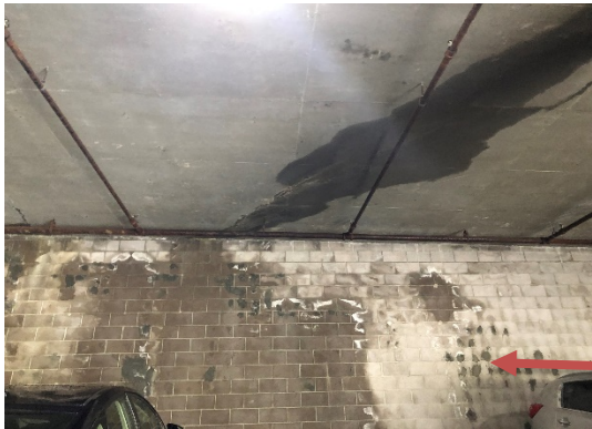
Fig 14 – Retaining Wall Patches
