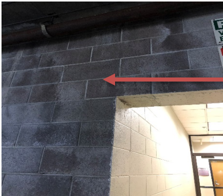
Fig 23 –No Diagonal Cracks in Masonry
