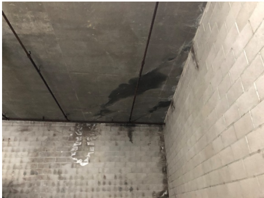
Fig 12 – Garage Masonry Walls
