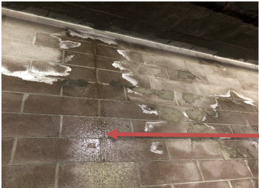
Fig 13 – Garage Retaining Wall
