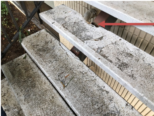
Fig 21 – Spalling of Exterior Stairs
