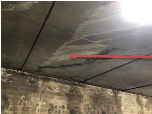
Fig 7 – Efflorescence Under Deck
