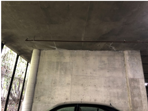
Fig 11 – Concrete Shear Wall
