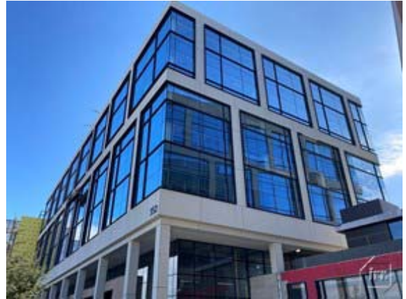
Phase I – Building B
