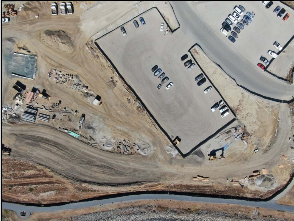
Above: Site Development Work
