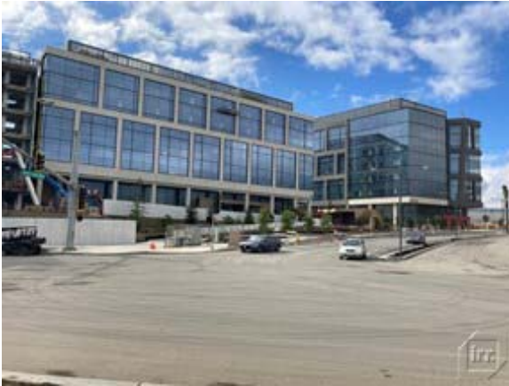
Phase I – Buildings B & C
