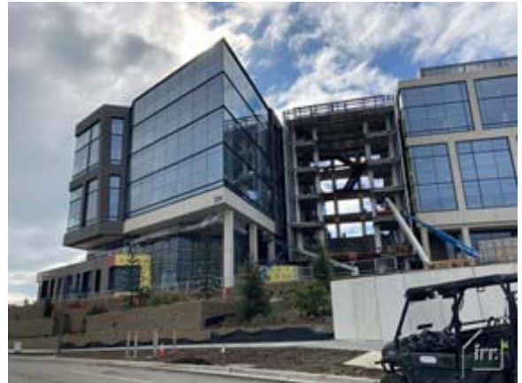
Phase I – Building A & Outdoor Meeting Space
