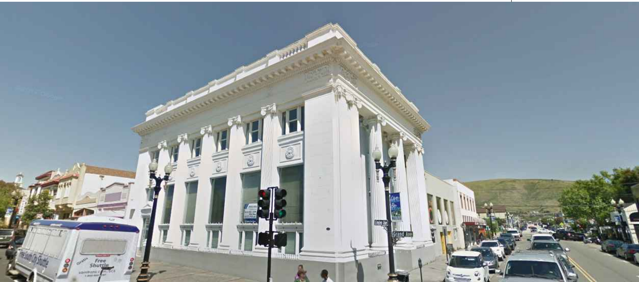
VIEW FROM LINDEN AVE AND GRAND AVE INTERSECTION
