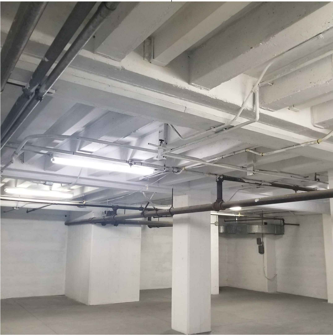
EXISTING BASEMENT INTERIOR
