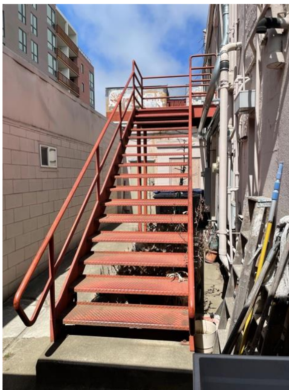
Back steps to office
