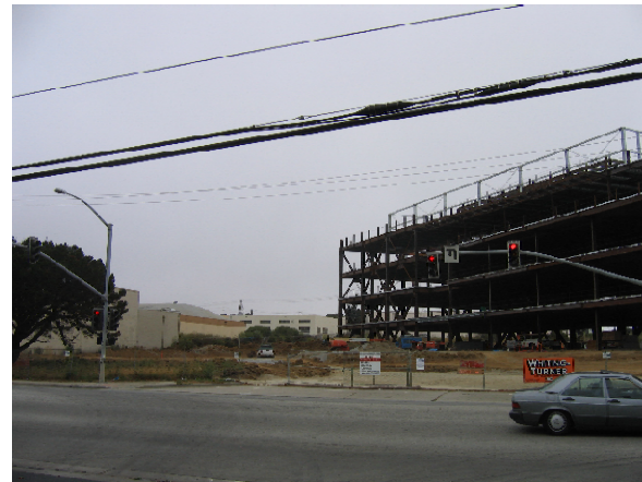
F New construction south of project site
