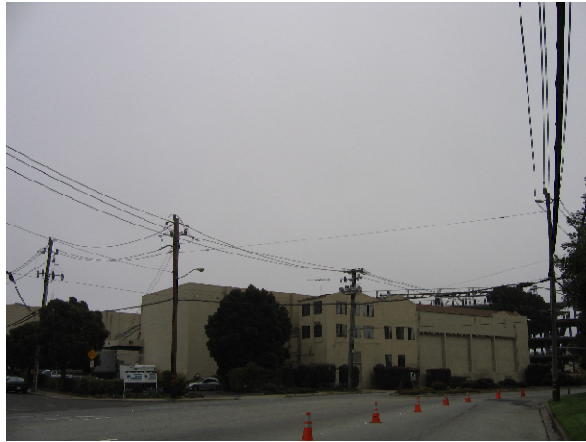
A Existing Warehouses on site
