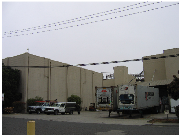
C Loading dock and Warehouses
