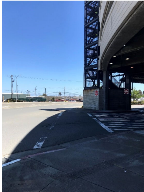
Pedestrian crossing along Huntington Avenue facing east where buses enter the SamTrans hub. Source: Fehr & Peers, 2021
