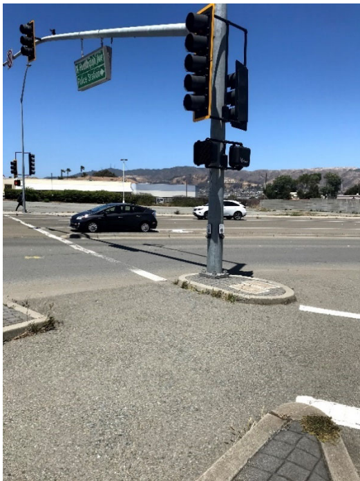
East leg crossing at Huntington Avenue and Sneath Lane facing north. Attention to the approximate 90 ft. wide crossing distance and the large pedestrian refuge island.
