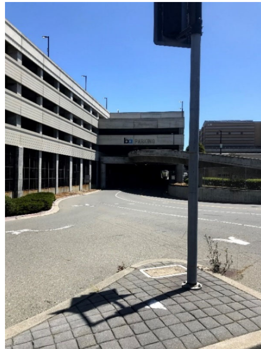
East leg crossing at Huntington Avenue and Sneath Lane facing south. Attention to the approximate 30 ft. wide slip lane and angle at which vehicles turning right will approach the pedestrian crossing.
