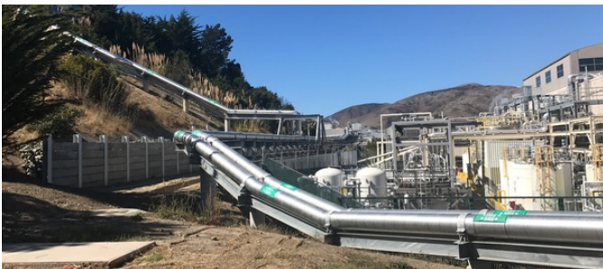
New Refrigerated Water & Glycol Piping at B3
