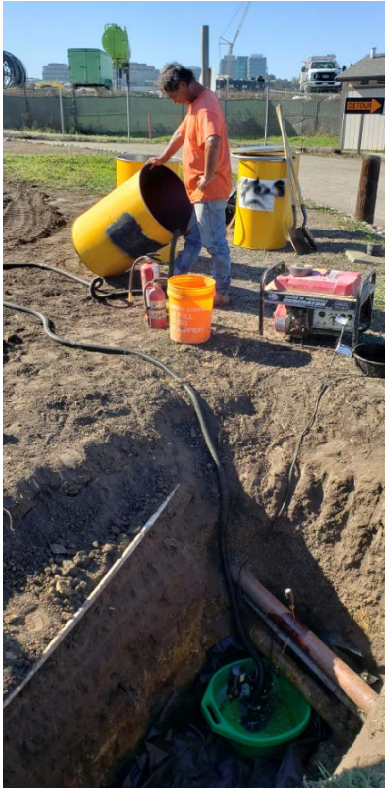
Draining fuel from underground fuel lines.
