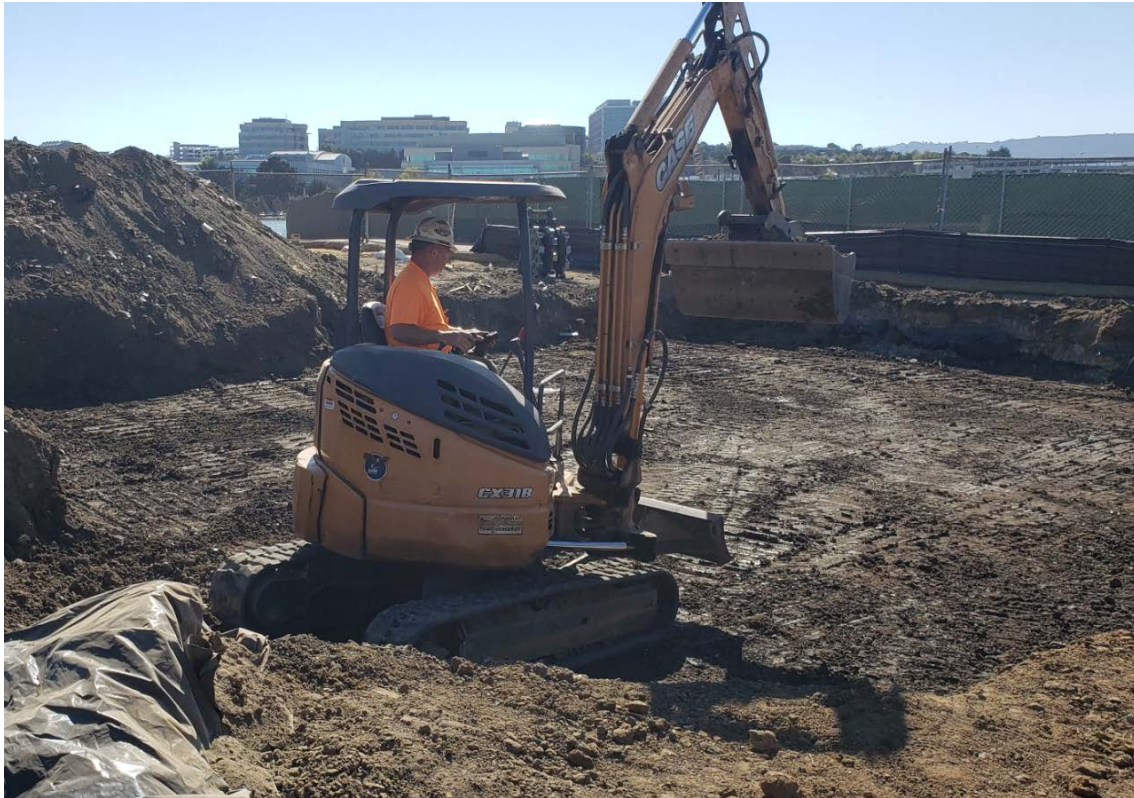
New clay cap material installed over tank pits.
