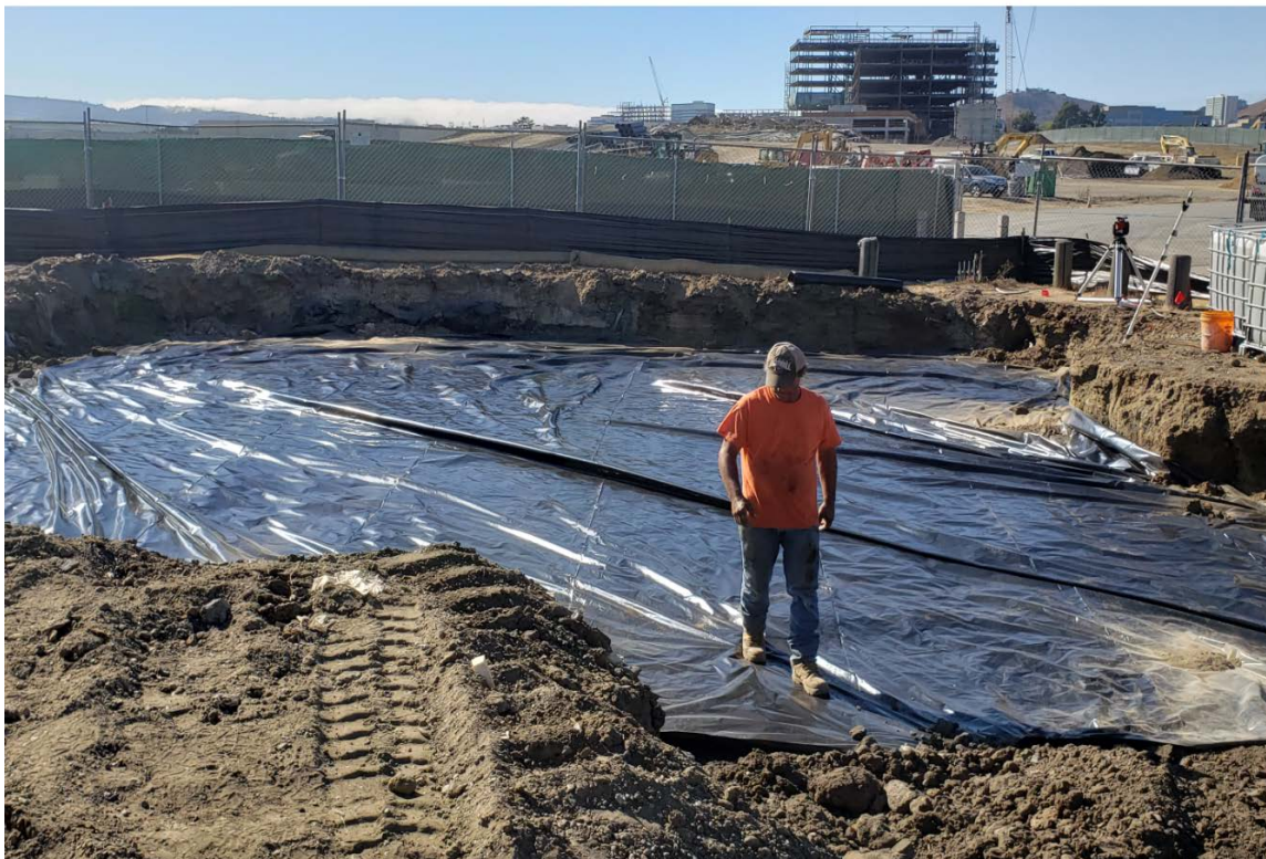
Installing a plastic membrane over the clay cap.
