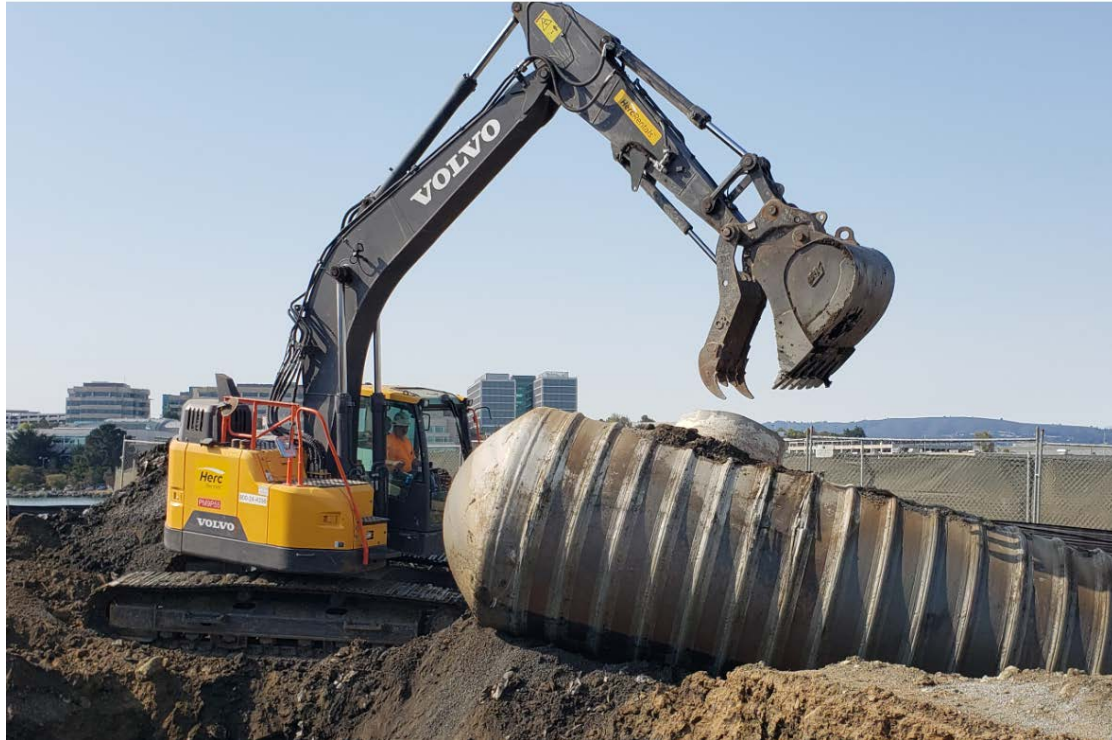
Removing fuel tank from Pit
