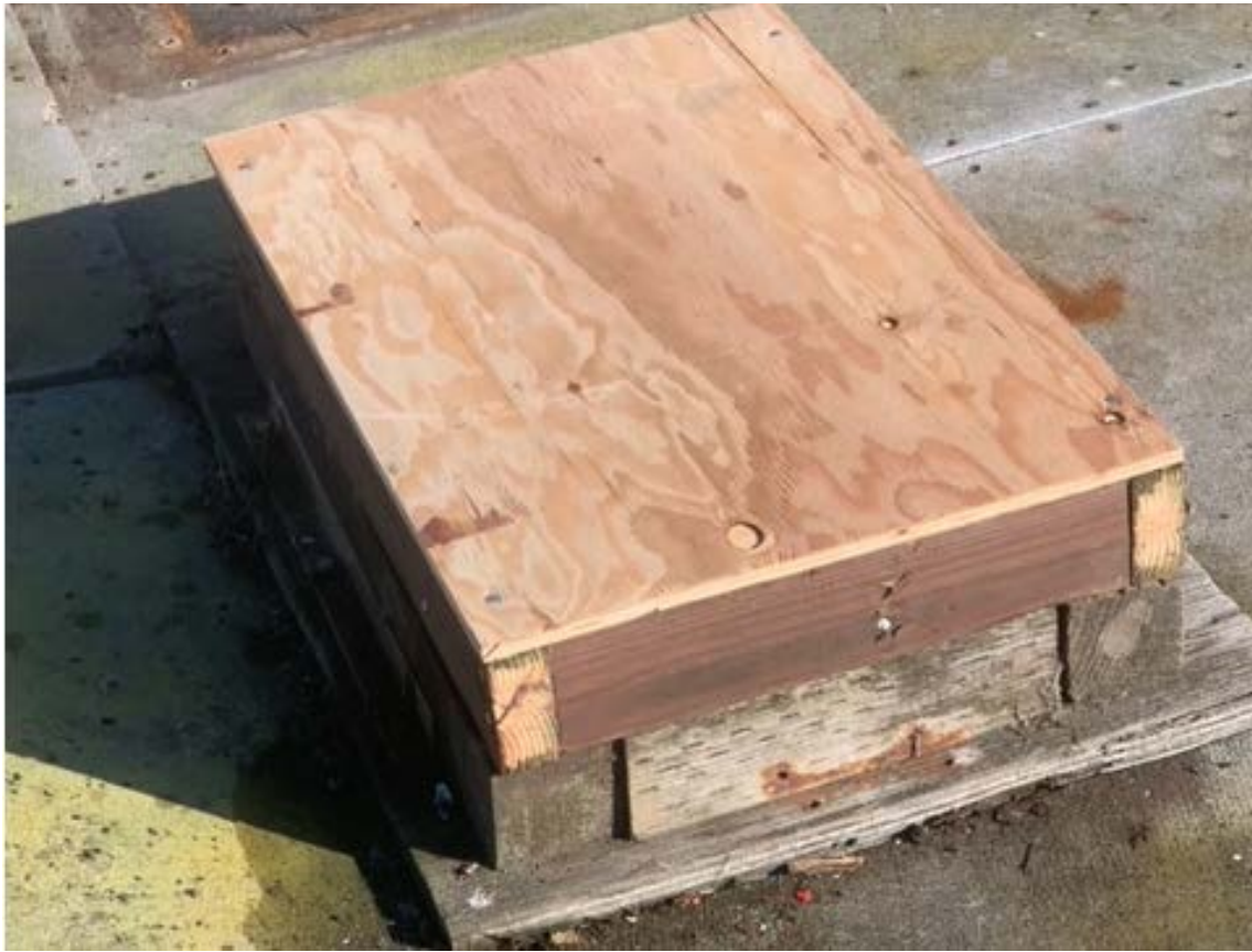
Dispenser pad on dock capped with plywood.
