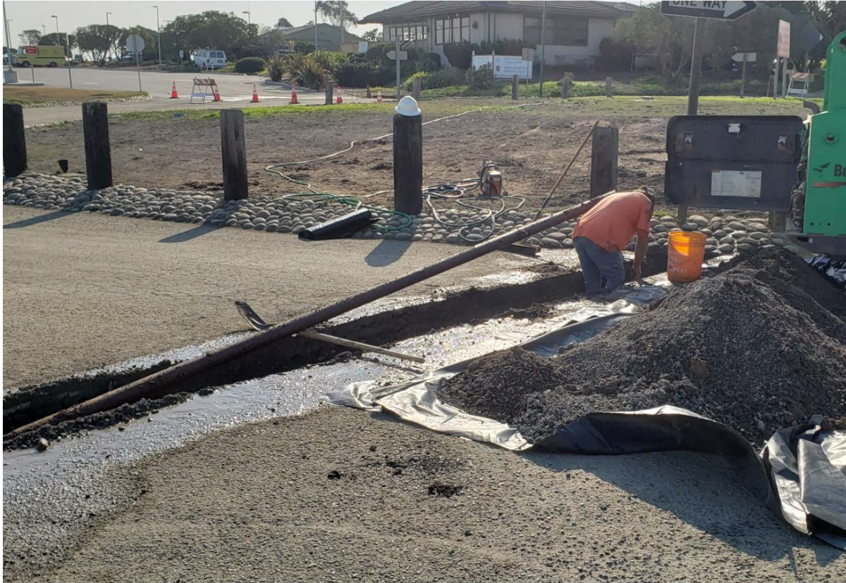
Removing a fuel line.
