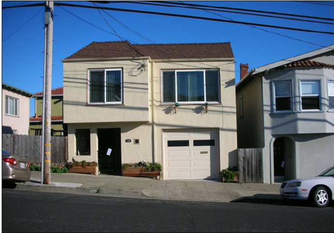
LEFT-SIDE NEIGHBOR FRONT ELEVATION - A 2-STORY SINGLE FAMILY BUILDING.
