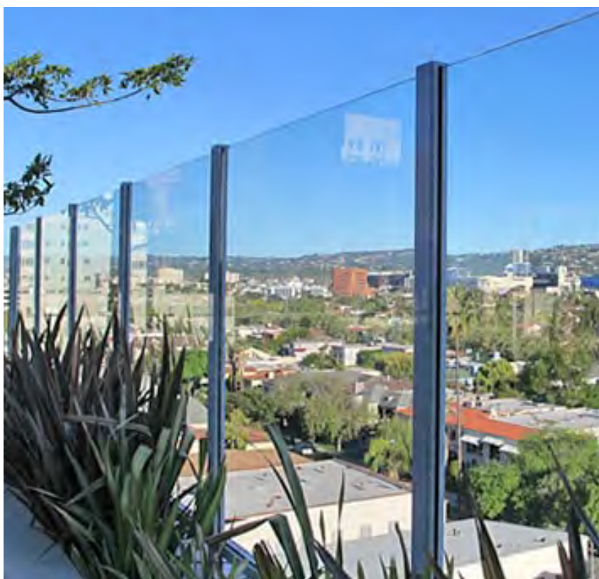
C1-3 GLASS GUARDRAIL
