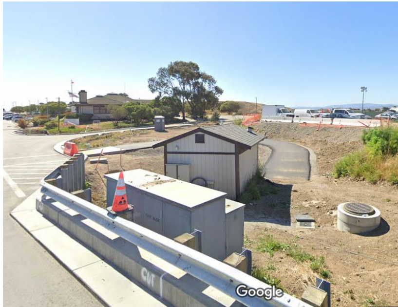
Existing Pump Station
