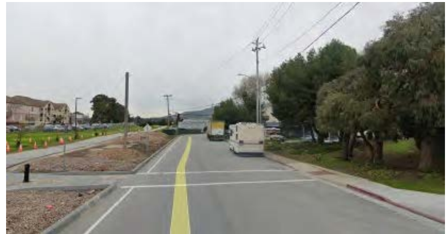
View North on South Maple Avenue
