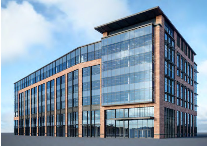
Building 7 - Northwest View
