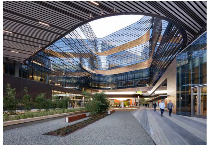
Example of a state-of-the-art commercial campus (Samsung North America Headquarters, San Jose, CA)
