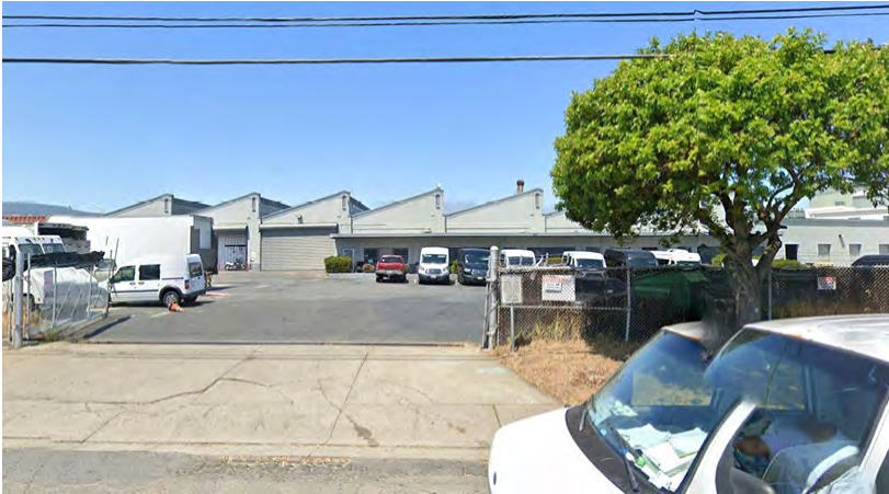
View West from Dollar Ave.
