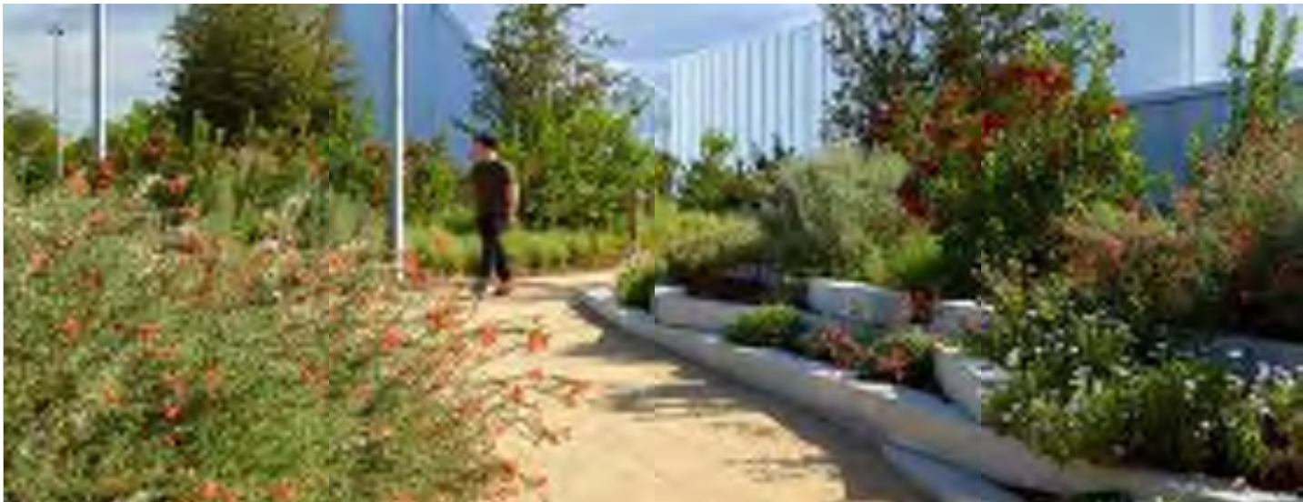
6 STABILIZED CRUSHED STONE PAVING
