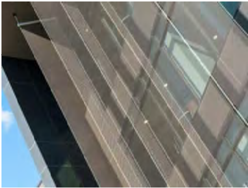
PARKING GARAGE FACADE AT ENTRANCES WITH (METALSCREEN MATERIAL)
