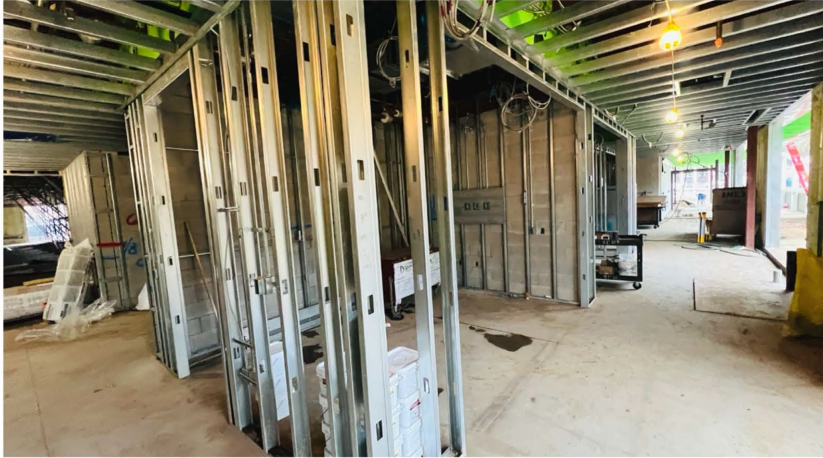
Interior framing and overhead rough-in nearing completion.
