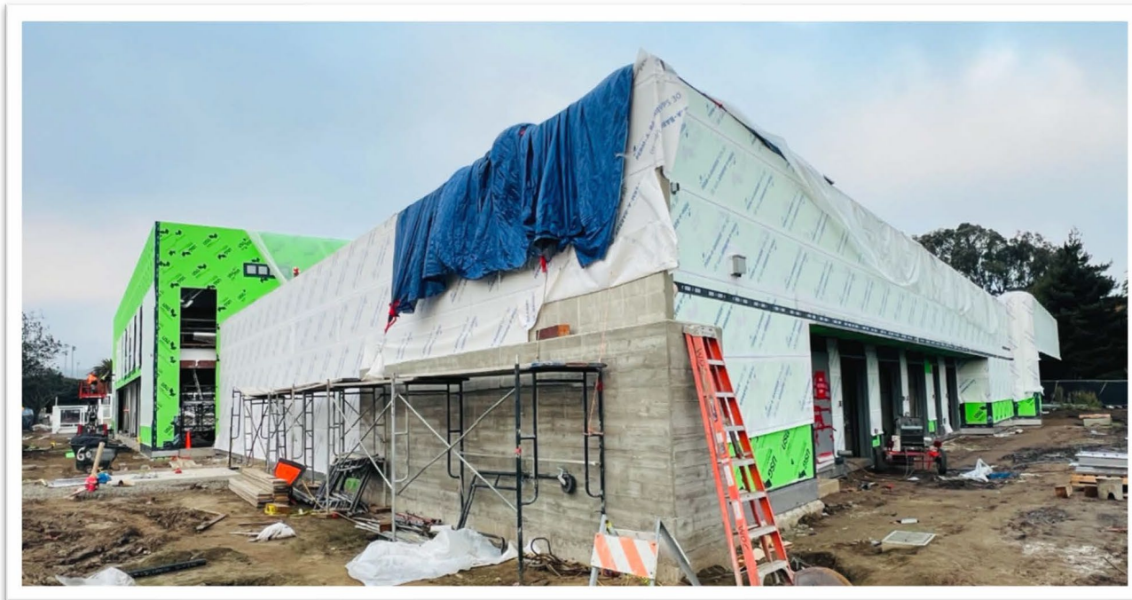
Sitewide view of building progress — envelope sheathing and framing in place.
