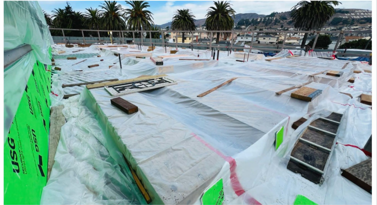
Roof preparation continues above the low roof in advance of waterproofing.
