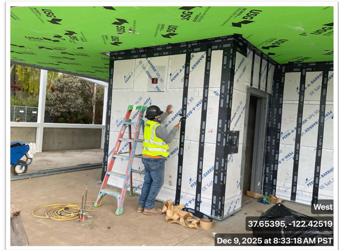
Air barrier installation in progress.
