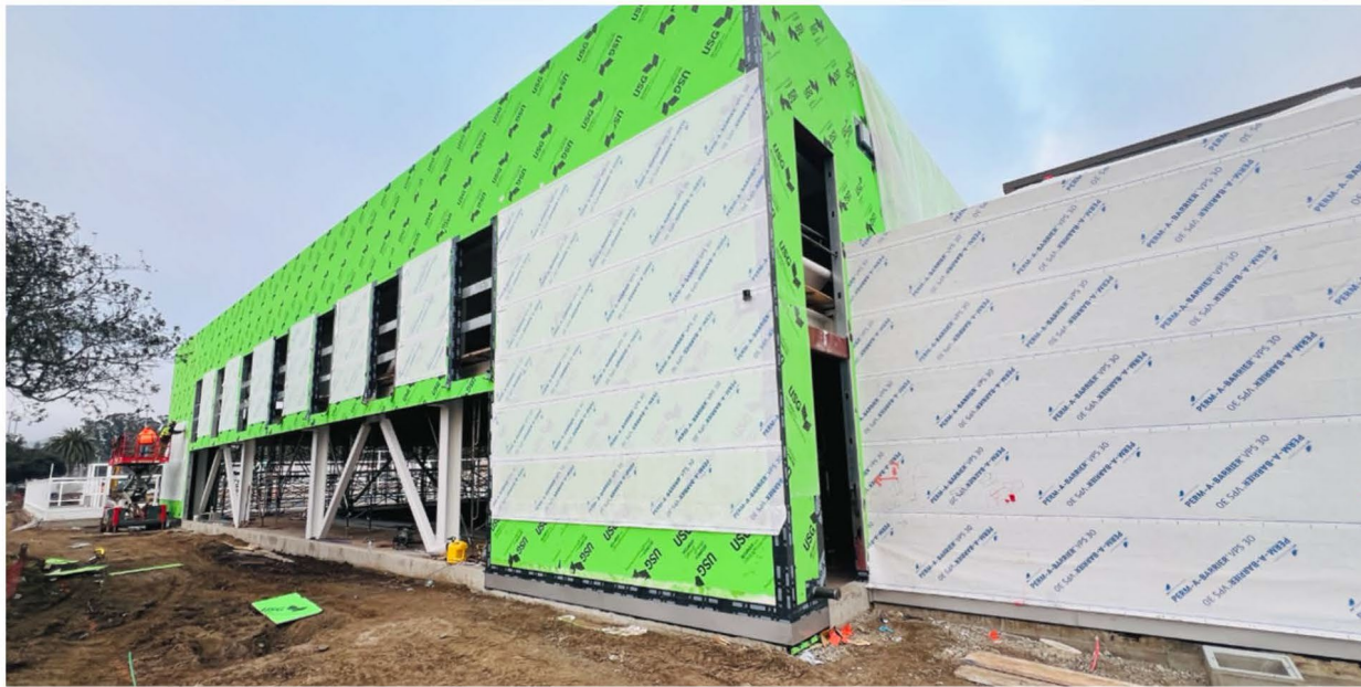
Air barrier installation in progress.
