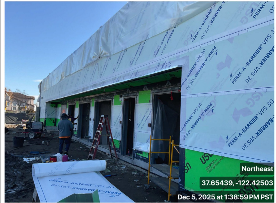
Air barrier installation in progress.
