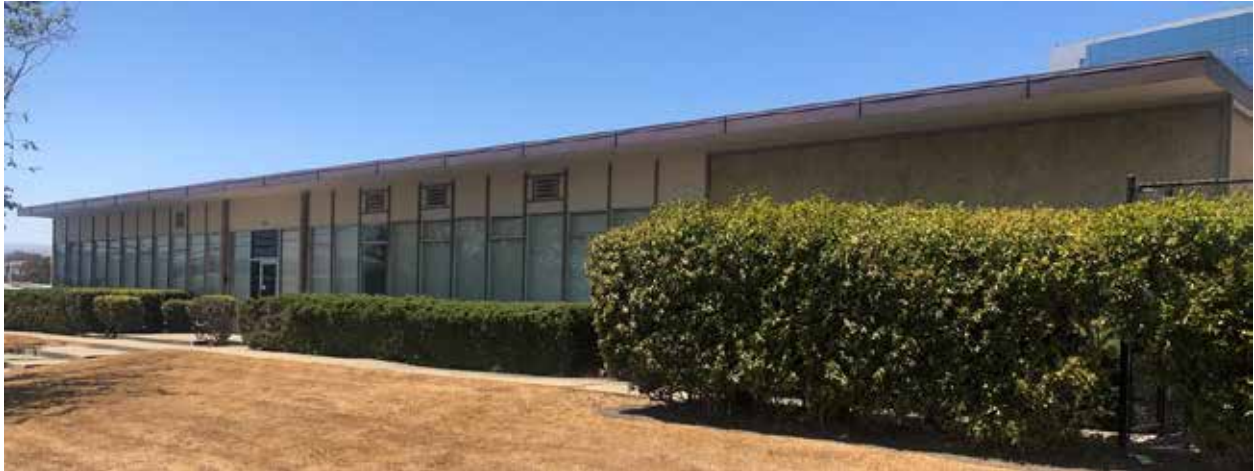
Fig.11 – 439 Eccles Ave. - Front looking west
