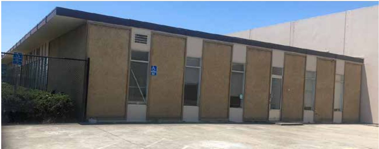
Fig.13 – 439 Eccles Ave. – Northeast side of office building
