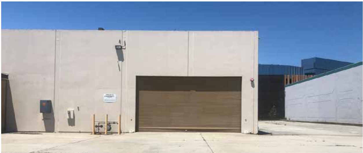
Fig.14 – 439 Eccles Ave. – Warehouse front, right side, looking northwest from driveway
