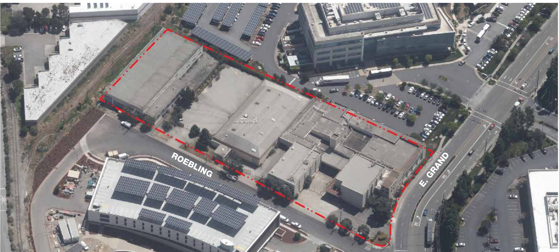
AERIAL VIEW OF SITE - WEST
