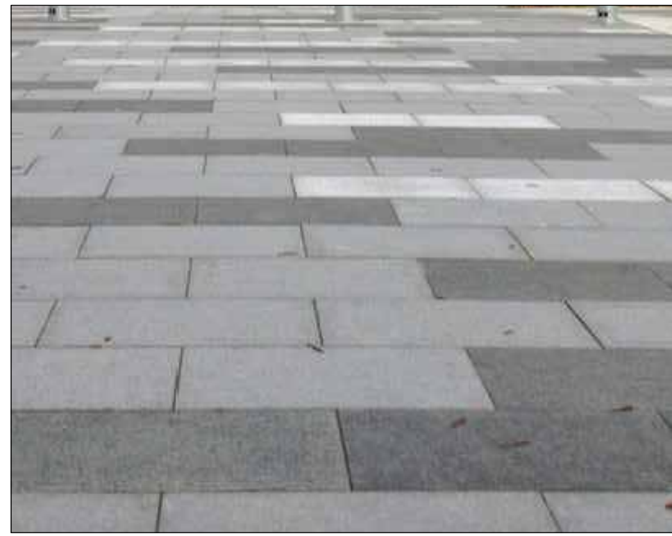
A NARROW CONCRETE UNIT PAVERS (PEDESTRIAN) MODEL: 12"X24" ACKERSTONE COLORS: MIX OF LIGHT, MEDIUM & DARK GREY
