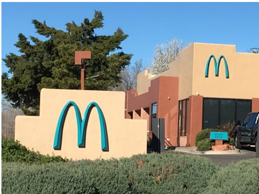
Figure 20.360.005.F: Example of a Freestanding Sign Incorporating the Architectural Details of the Main Building
