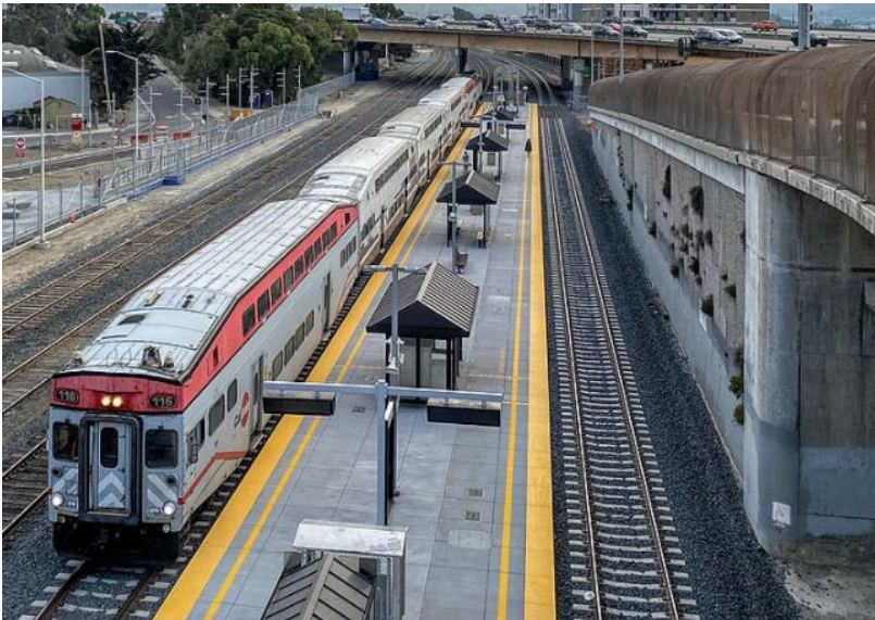
Rendering of the New Widened Central Platform at the South San Francisco Caltrain Station
