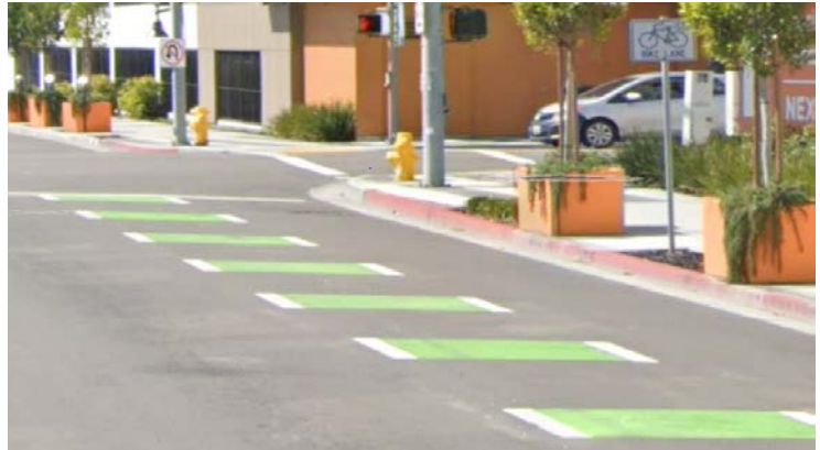
Class II Bike Lane on Airport Boulevard
